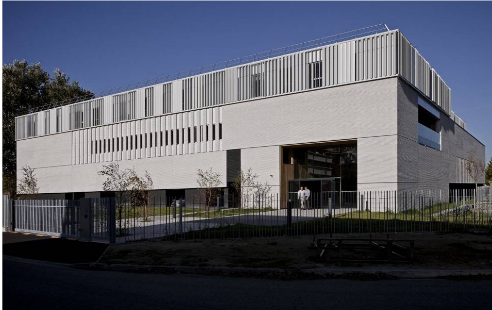
Figure 14 : CLS Toulouse new building
