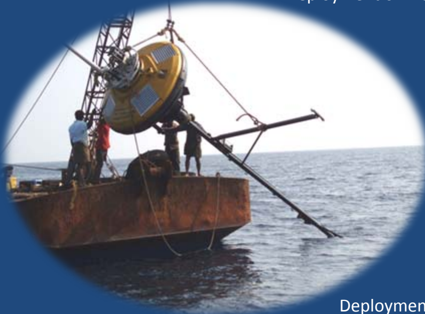
Deployment of Met – Ocean buoy
