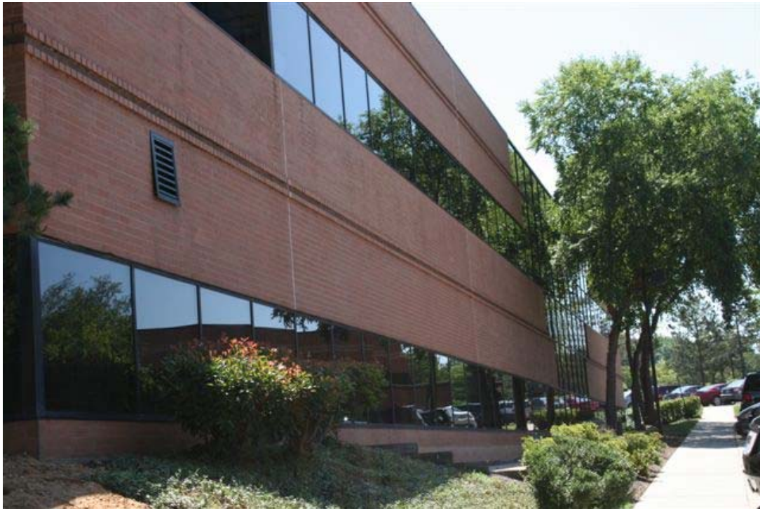
Figure 22 : CLS America new building
