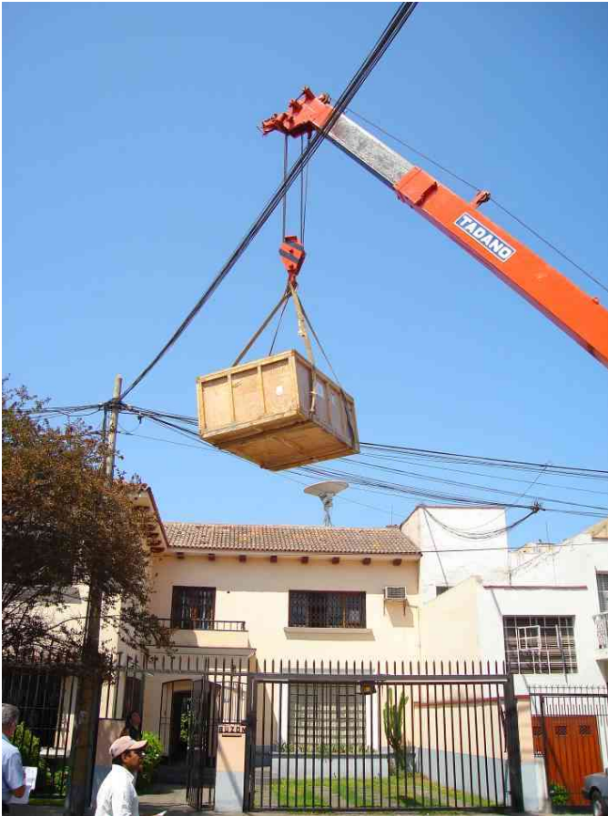
Figure 14: CLS Peru Regional Processing Center
