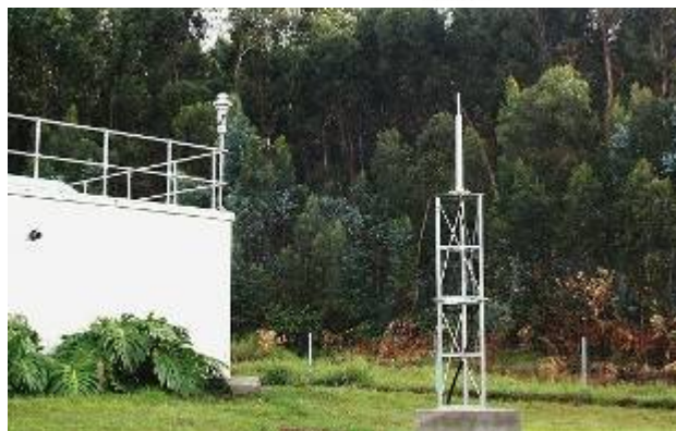
EXISTING CNES DORIS ANTENNA ON EASTER ISLAND
