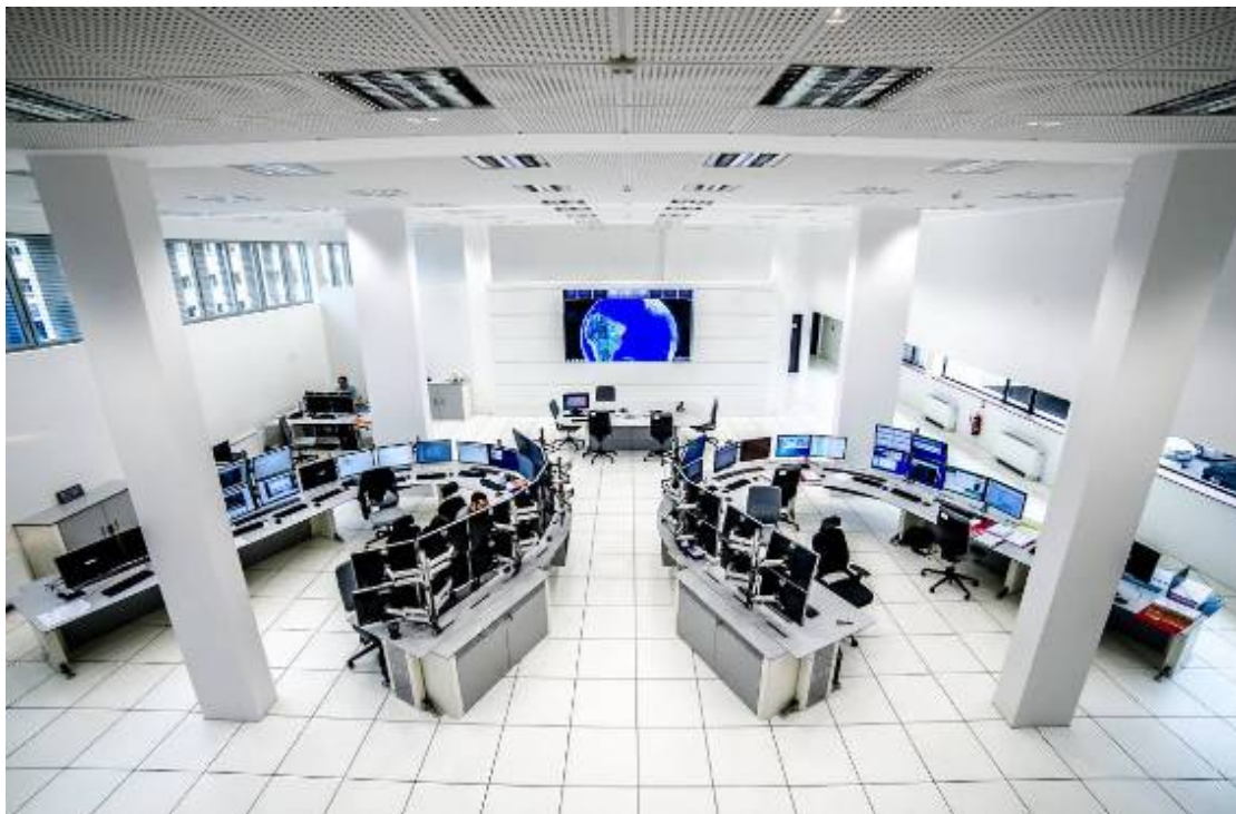
Figure 23 : CLS Toulouse Control Room
