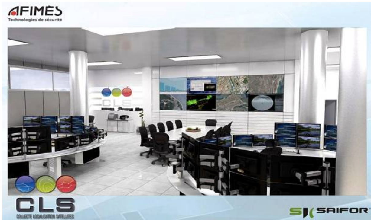
Figure 29 : New CLS control and monitoring room
