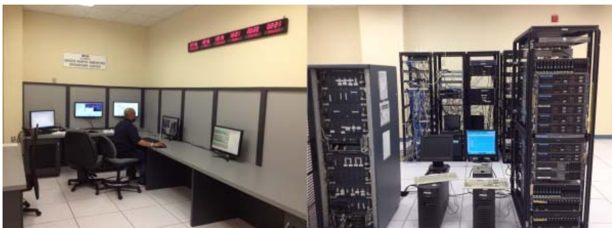
Figure 28 : CLS America Global Processing Center
