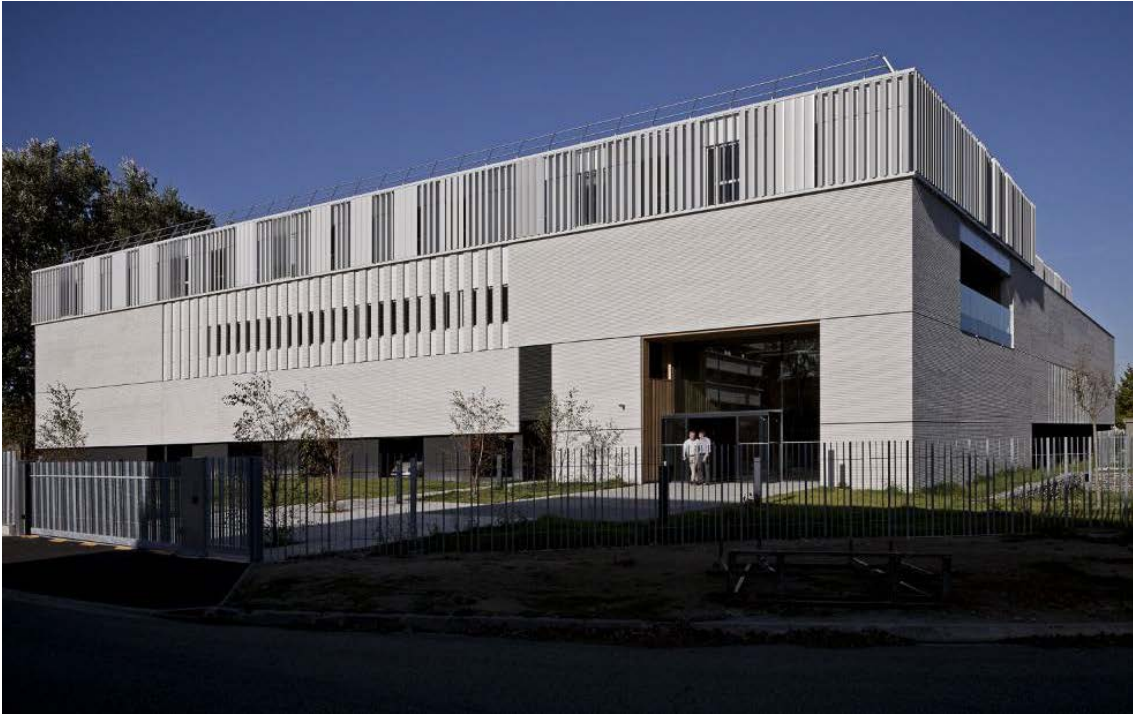
Figure 21 : CLS Toulouse new building
