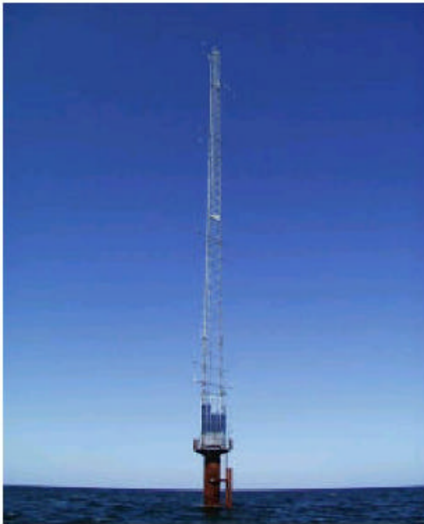
60m measurement station at Horns Rev, Denmark
