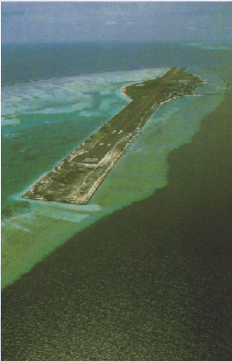
Maldives Int. Airport
