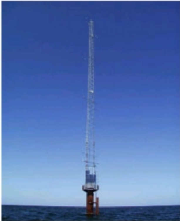
60m measurement station at Horns Rev, Denmark
